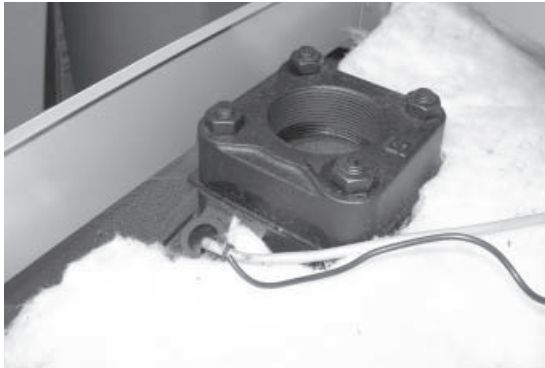
Fig. 13.16: Insertion of the probes into the sheath
